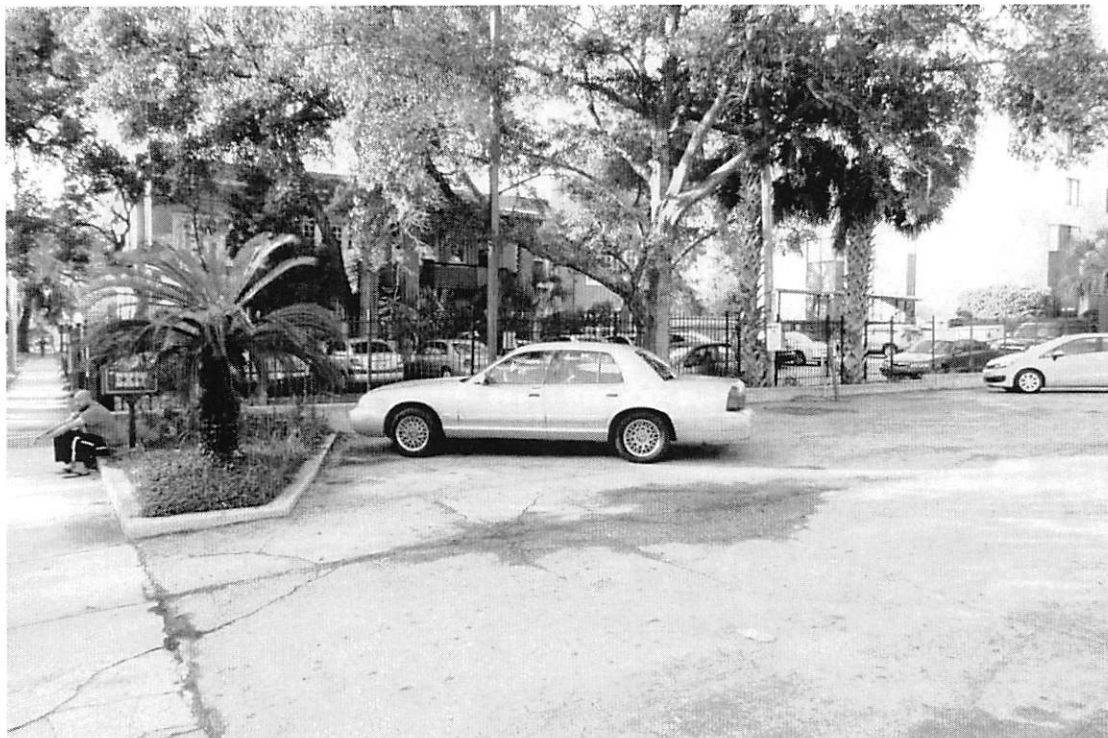
Parking area along south property line
