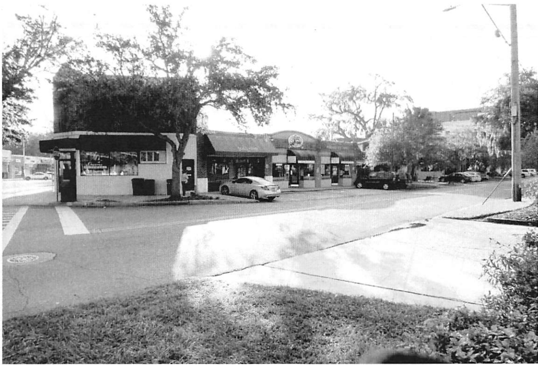
Commercial uses across Margaret Street.
